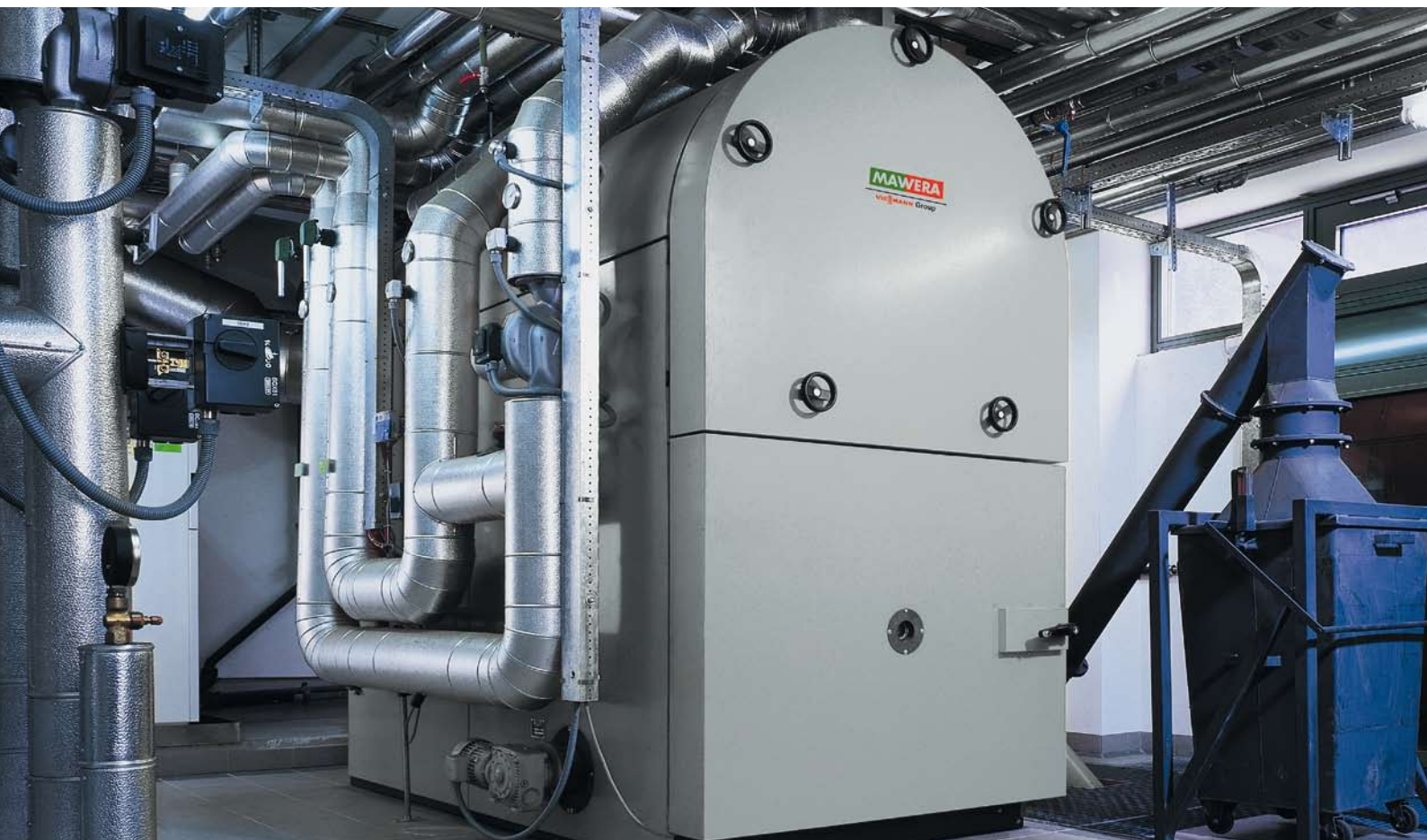
2 x palenisko podsuwowe FU 2500 RA, Mosser Leimholzbau, Randegg, AT
